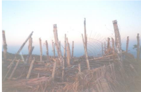
What remains of Bhujulichuk Meditation Centre after destruction by army personnel
